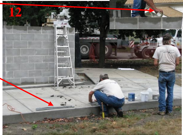
View of the epoxy preparation and application.
