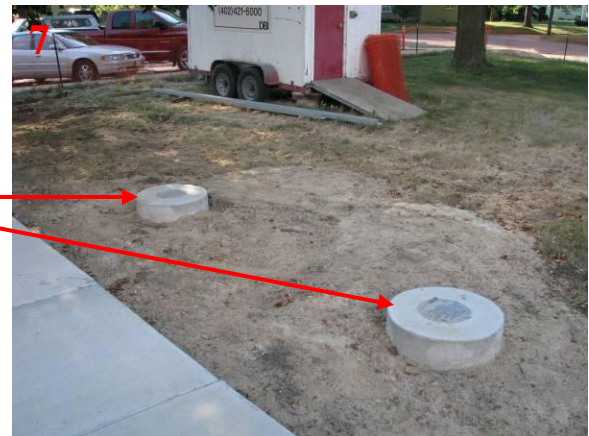
View of the flag pole bases north of the memorial.
