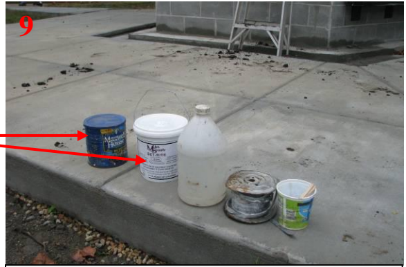
View of the epoxy products used to set the obelisk.
