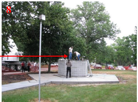
View of the obelisk foundation being prepped for the granite.
