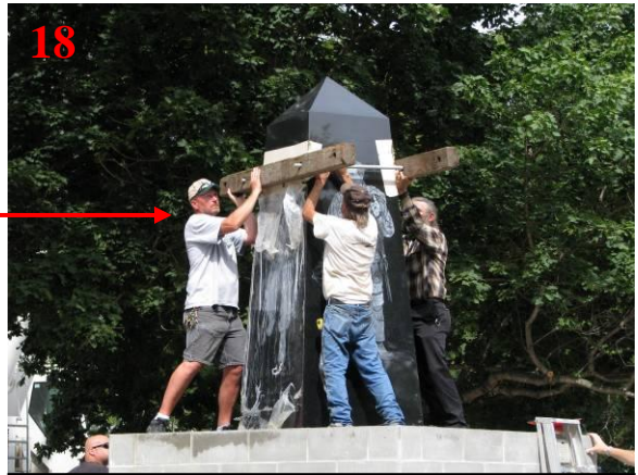
View of the crew removing the clamp from the obelisk.
