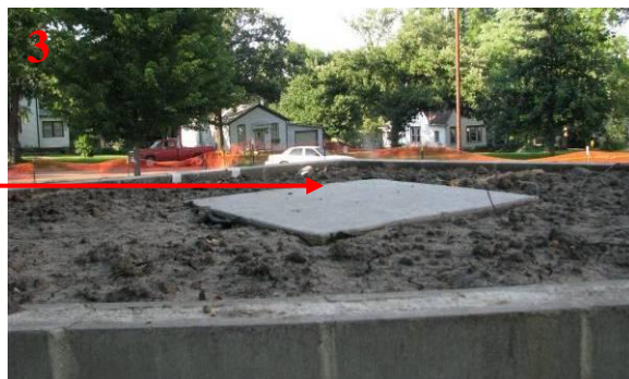
View of the obelisk base on the top of the memorial.
