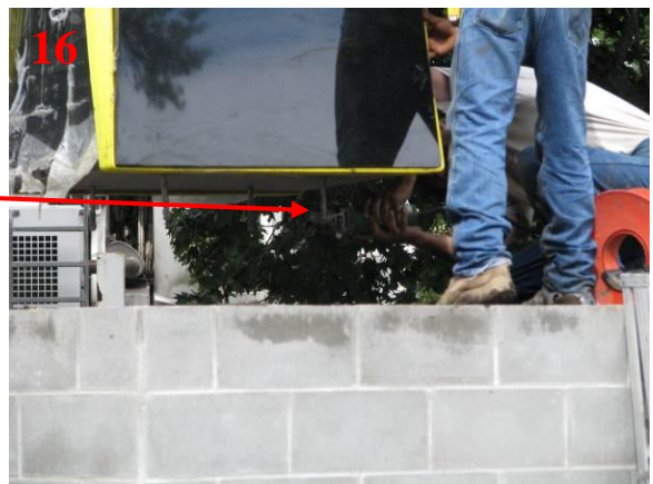
View of the workers cutting steel pins under the obelisk.
