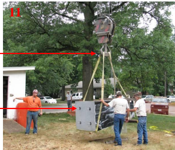
View of the obelisk being lowered prior to tipping it upright.
