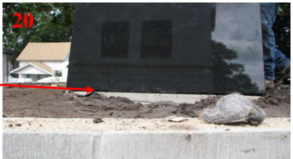
View of the obelisk where it sits on the concrete foundation.
